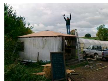
The newly re-roofed yurt
