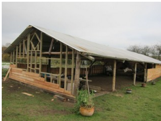
Hub-to-be! Early work underway
