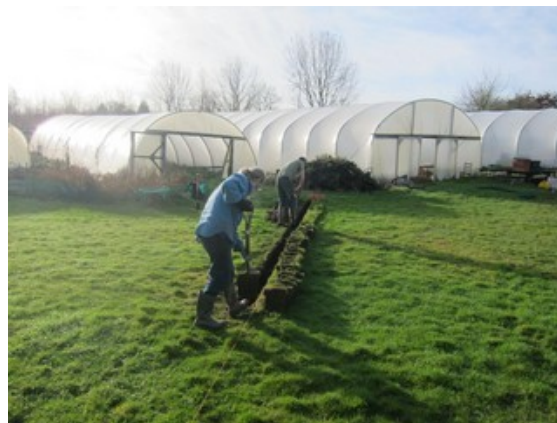
Drain digging in the social area
