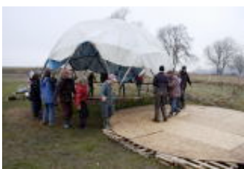
Moving the geodome onto its new platform
