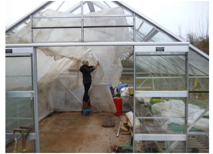
Bubble-wrapping the greenhouse to insulate it for 2017 seedling raising
