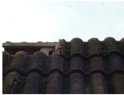
Roofer at work on the re-positioned shed
