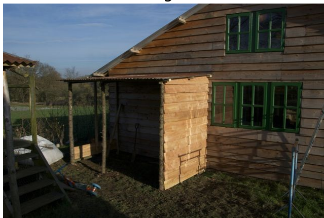
The new lean-to wood store
