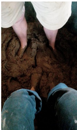
Preparing the render
