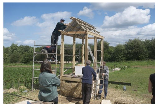
The tree-bog – construction well underway!
