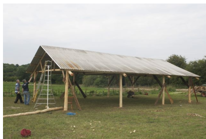
The completed barn
