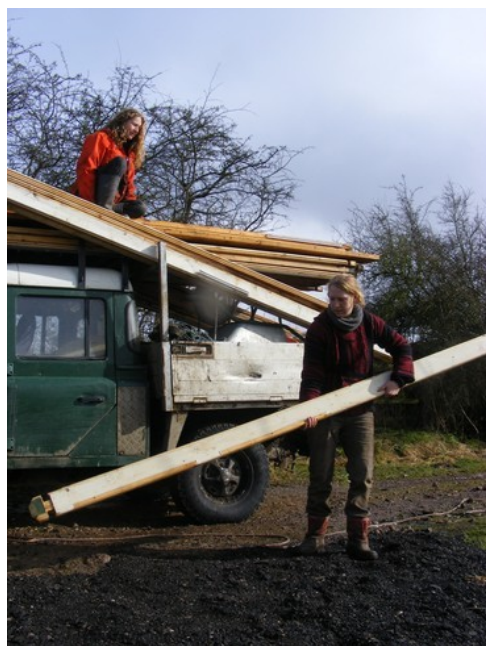
Building parts arrive on site
