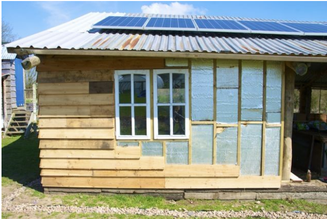
The new veg collection area in mid April
