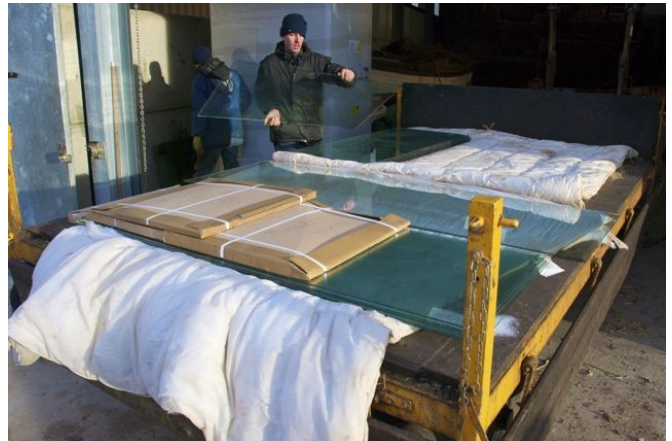
Unloading the parts for the new glasshouse
