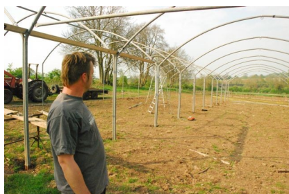
The frame for the new polytunnel
