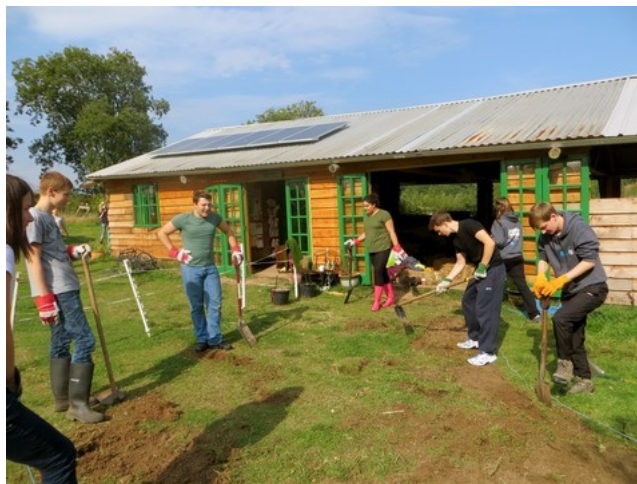
Challengers digging the path into the pole barn, including the challenge of digging earth that is like concrete!
