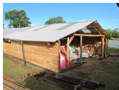
The pole barn extension
