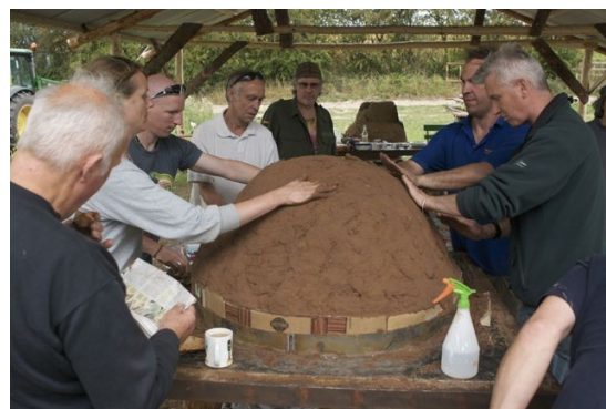
Applying the cob
