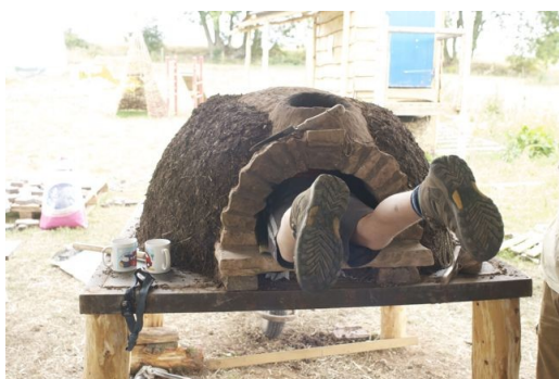
The perfect sized person for sweeping out the sand from the mould!
